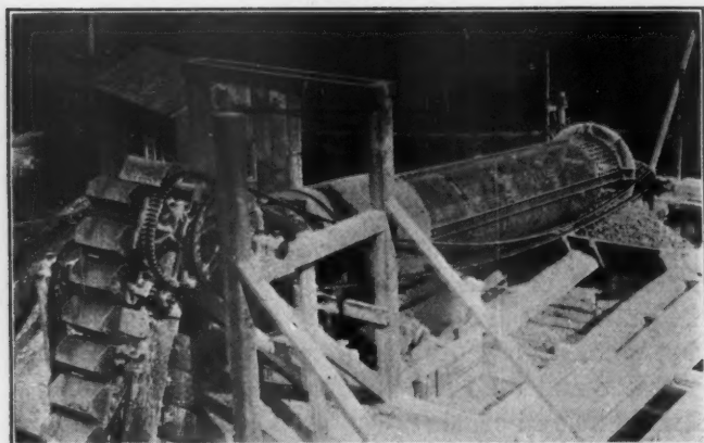
Bucket Elevator Head and Revolving Screen Over Bins
